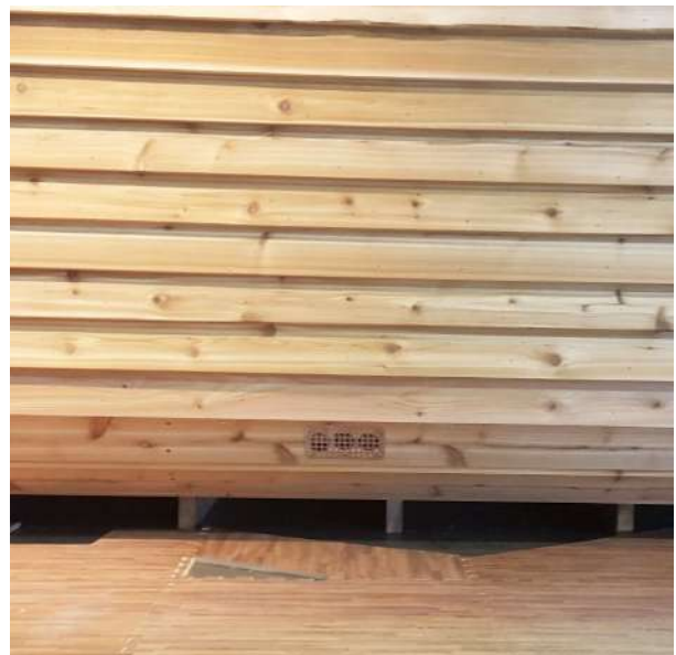
Inlet Vent on side wall under heater (outside)
